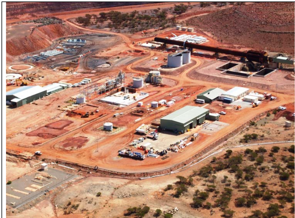
Windimurra Construction Site in Early April
