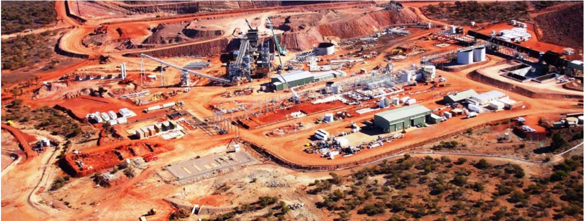
Windimurra Construction Site in late June
