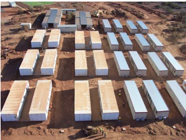
Construction Village being built at Windimurra March 2007
